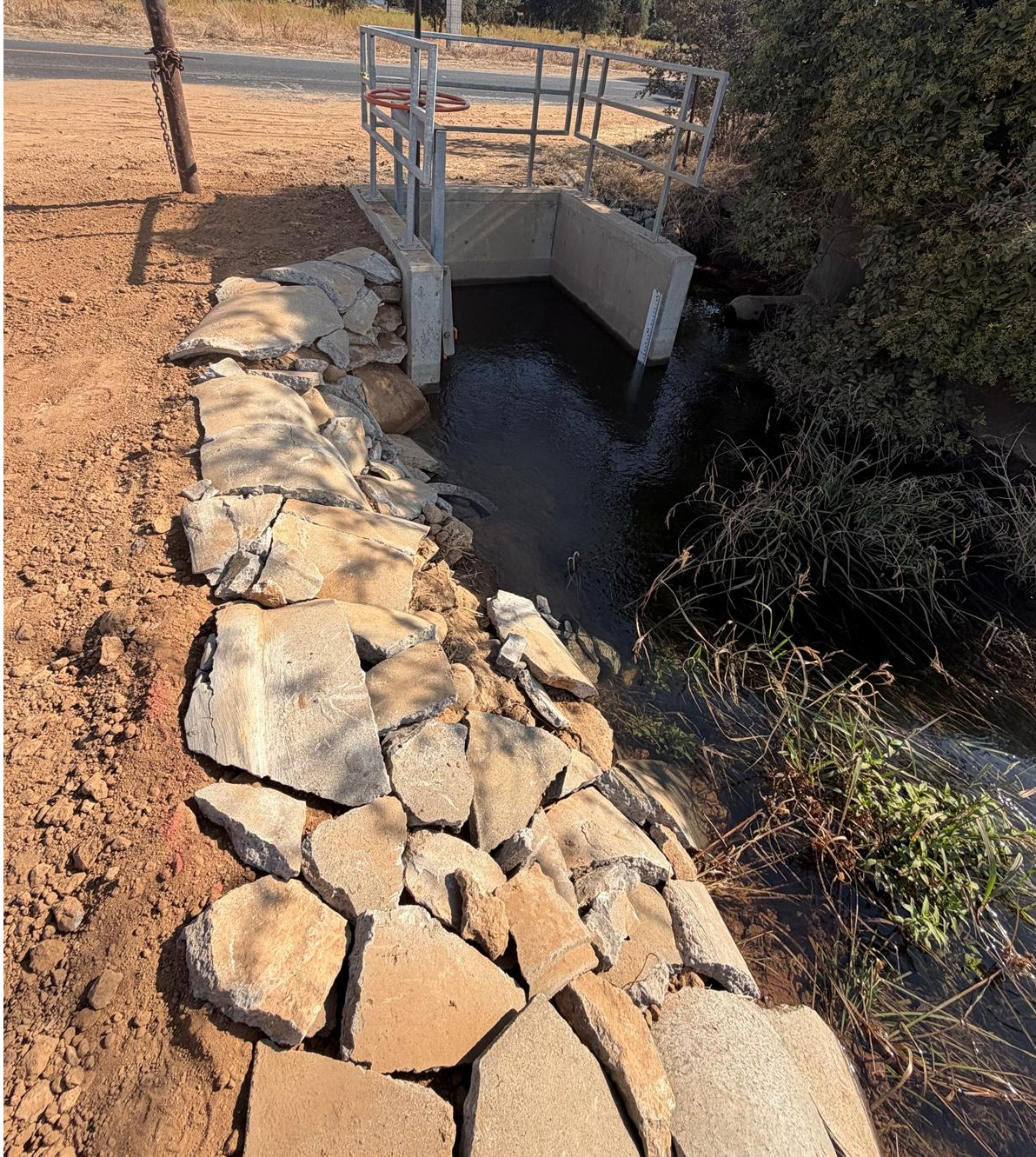
Staff asked Arnaudo to reuse some of the broken concrete to line the outfall to the East Ditch which had been undercutting the outfall wall
