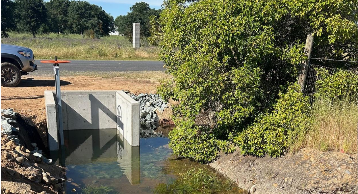
Operating Outfall on the East Ditch Near Brandt Road
