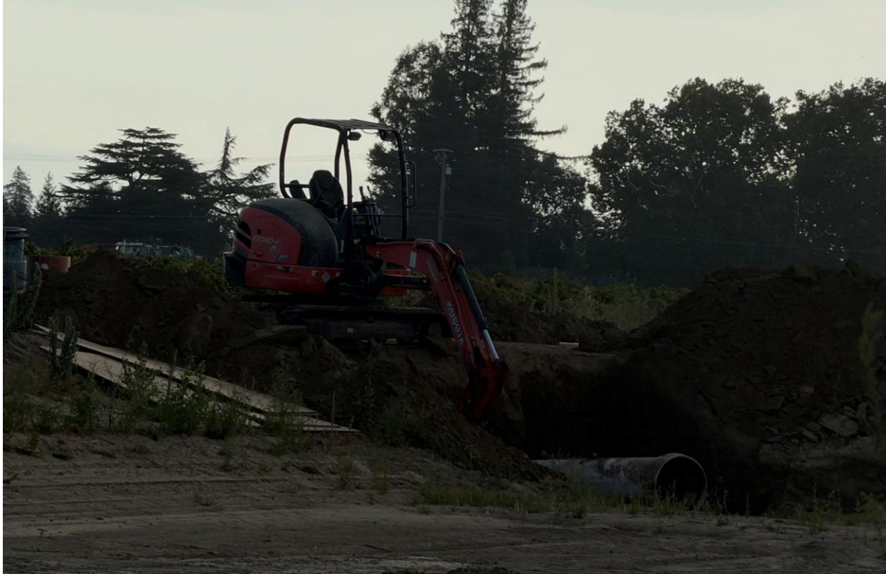
Central is back out at Teck Basin installing the outfalls
