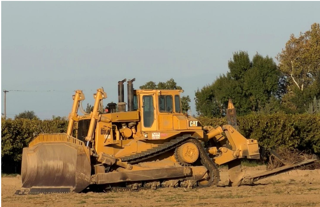
D10 staged to rip Locust Tree basin
