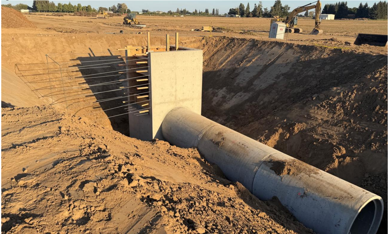
The structure at the toe of Locust Tree basin under construction
