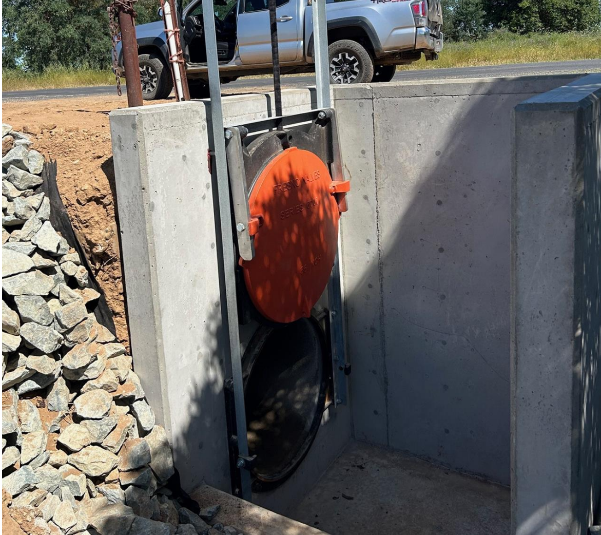
Finished Outfall on the East Ditch Near Brandt Road
