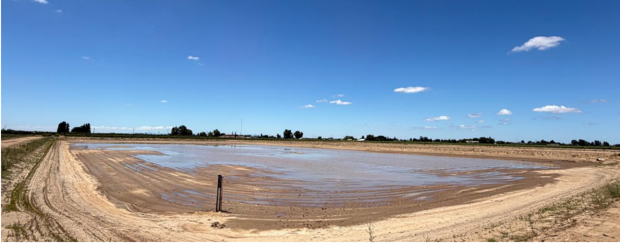
The Eastern side of Teck Basin is finally nearly dry!
