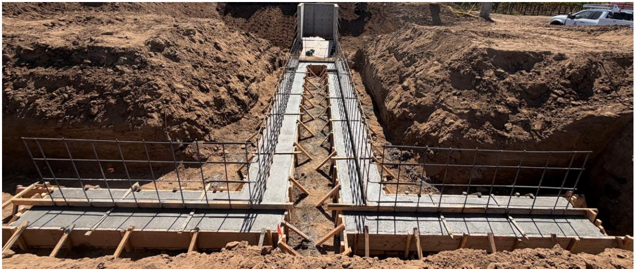
The structure at the toe of Locust Tree basin under construction
