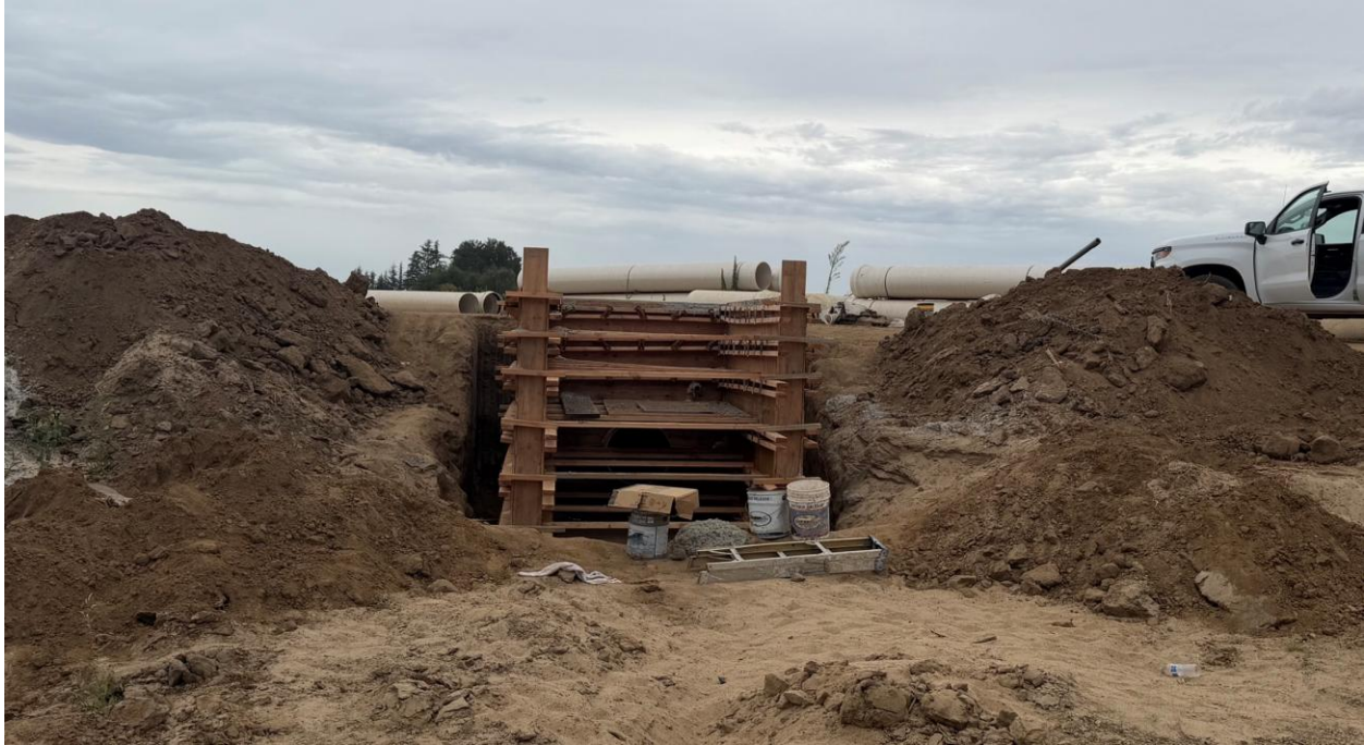
New Teck Basin east outfall was poured on Friday
