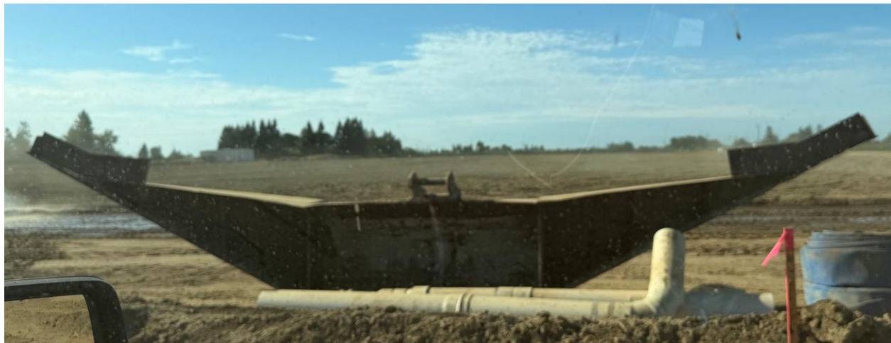
Lidco tile drain installation near Teck Basin
