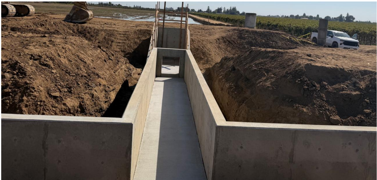
The structure at the toe of Locust Tree basin under construction
