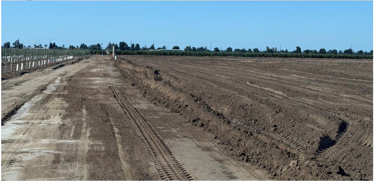
The Locust Tree East Levee arising from the farm road
