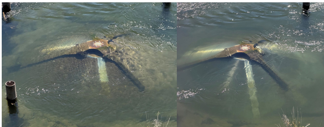
South Screen before and after a hand cleaning
