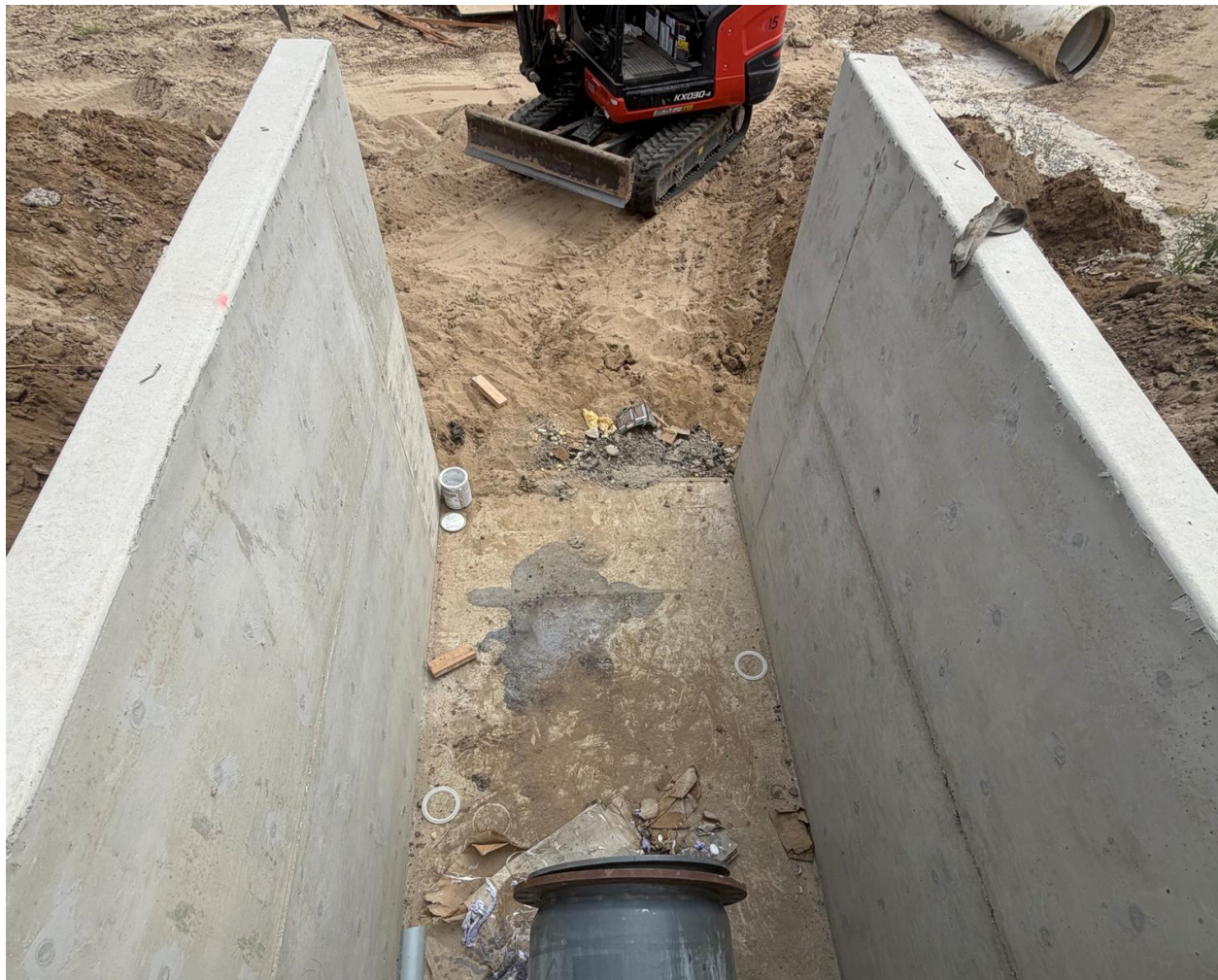
Teck Basin outfall
