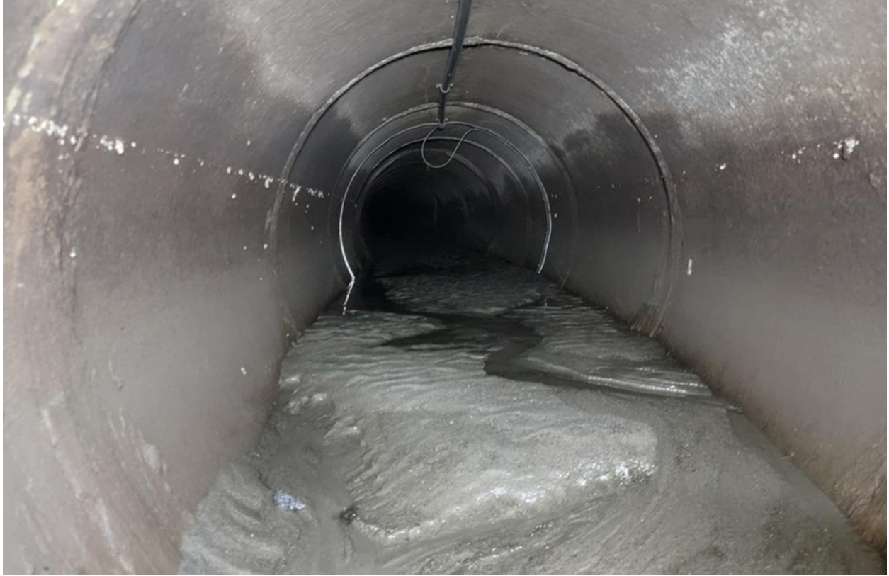
Brandt Road Extension Lateral
