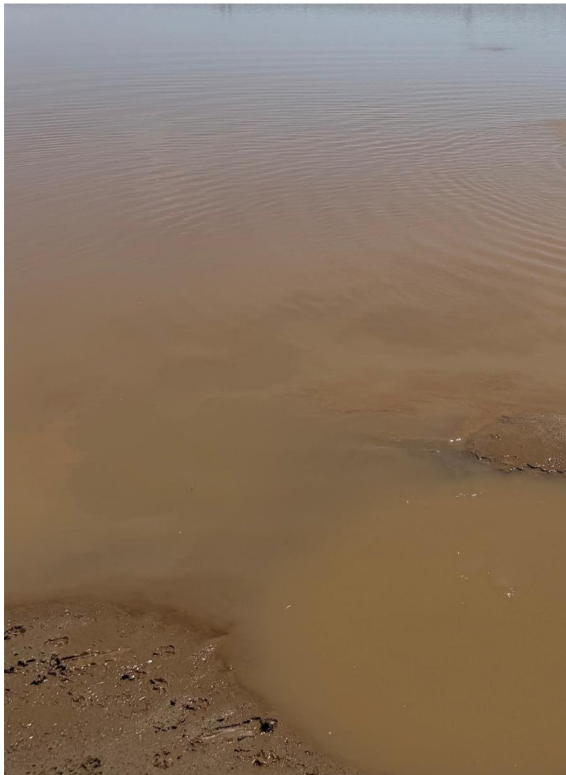
Boils coming from an old low head line foil efforts to drain the East Basin
