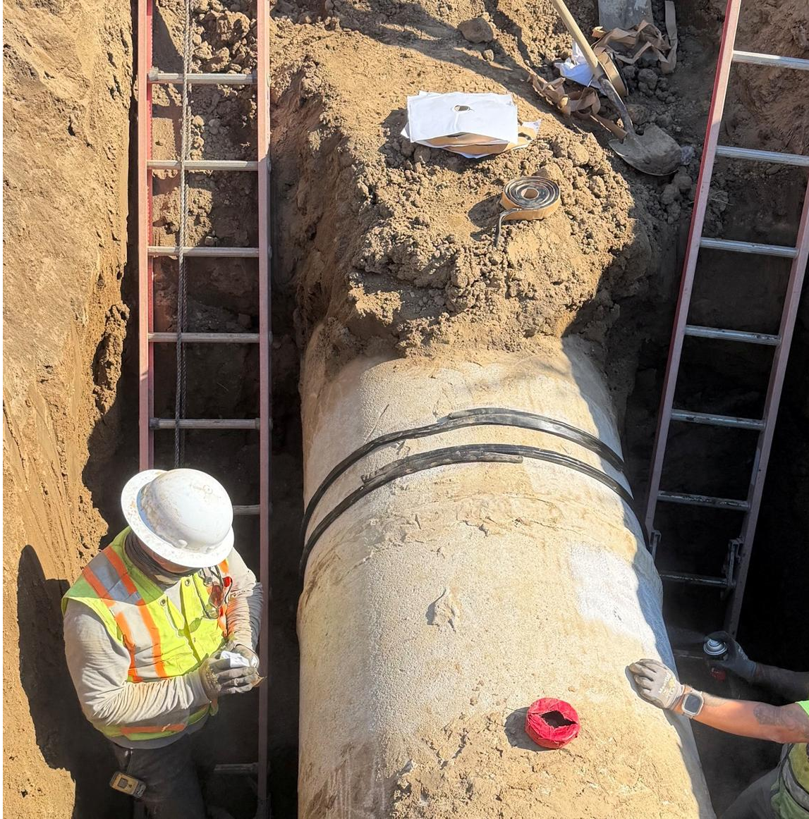
SS Main Repairs on Tretheway
