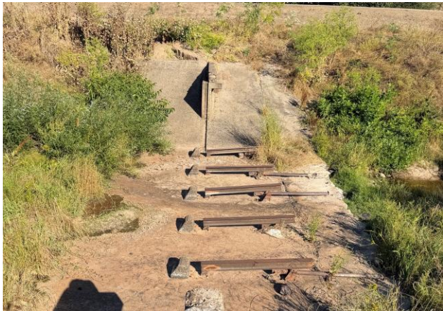
Lockeford Springs Dam dry
