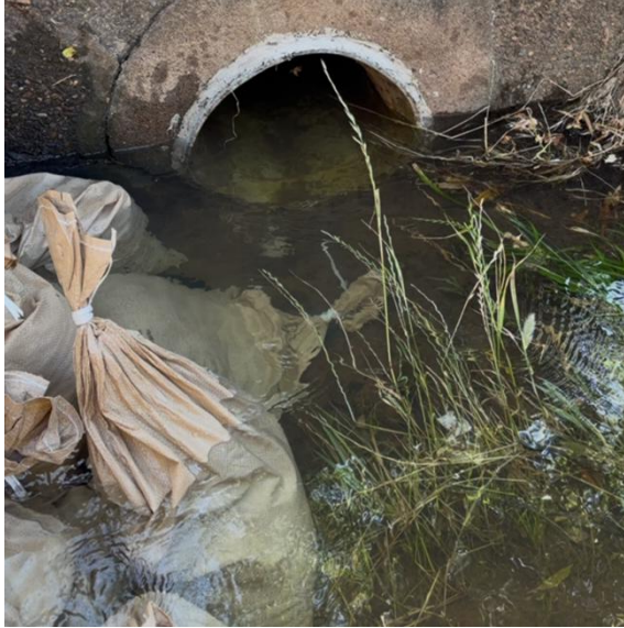
East Ditch Dam and lateral
