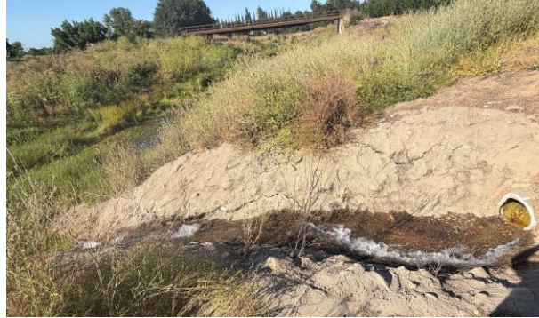
2 nd District Outfall into Bear Creek above the dam
